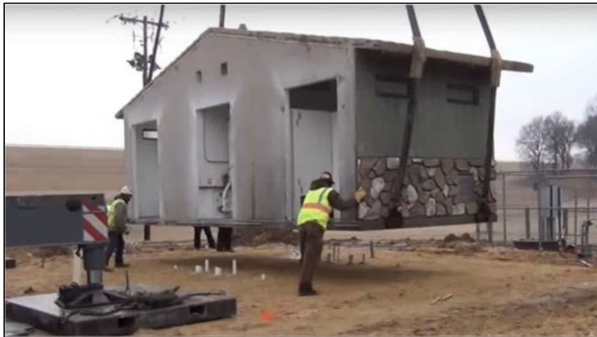
Figure 23: Placement of CXT Unit [7][8]
