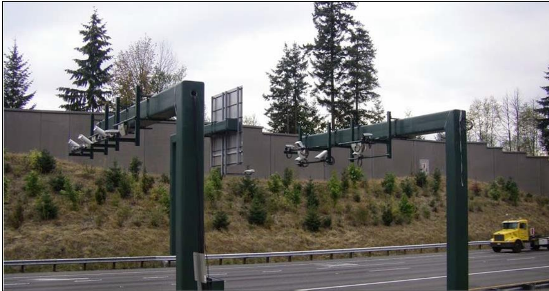
Figure 1: Gantry for Tolling System [13]
